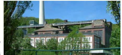
Cuno-Kraftwerk, Herdecke, Germany Natural Gas / 3.9 MW / 2 units
