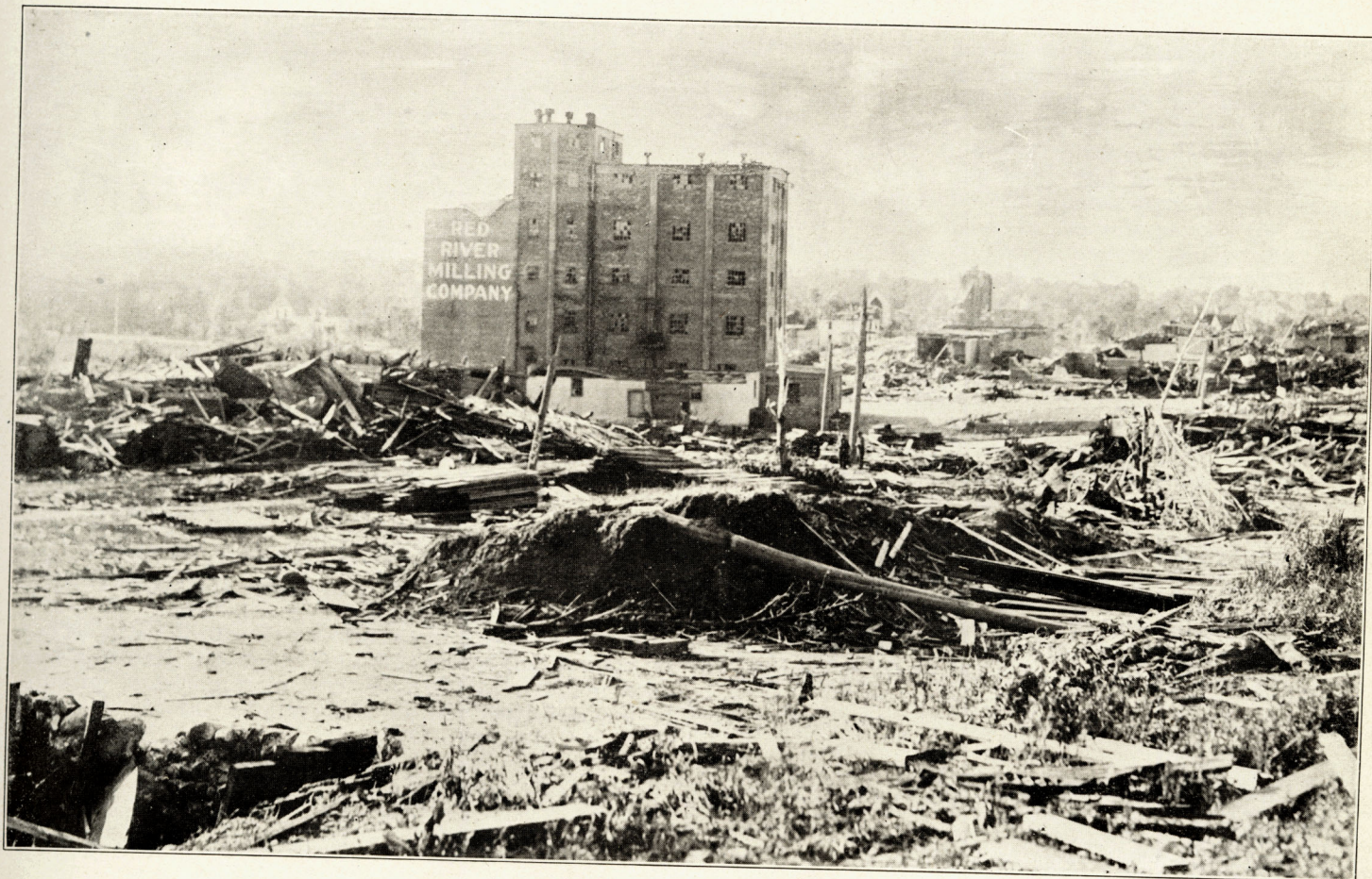
FIG. 2.—Tornado destruction along Red River in Fergus Falls, Minn.
