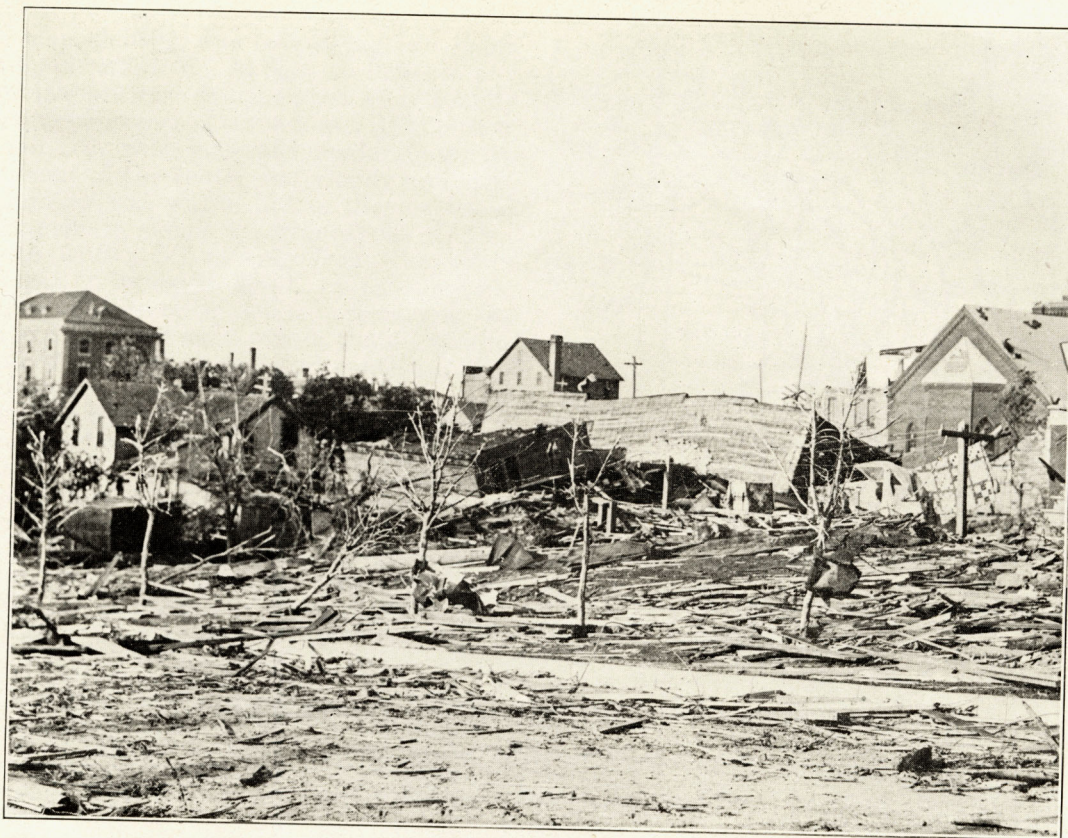
FIG. 1.—View of tornado damage in Fergus Falls, Minn. Note the trees stripped of bark, probably by the explosive action of the air in the bark, as the low pressure of the tornado passed. (Courtesy, Minneapolis Journal .)
