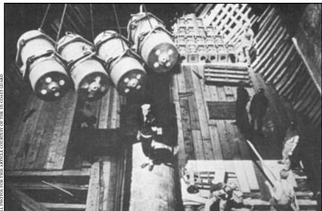
A member of an Explosives Loading Detail monitors the loading of high explosives and the work of carpenters as they construct the bombs' wooden framework in the ship's hold.
