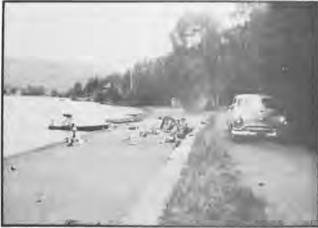
The beach, before the road was moved back.
