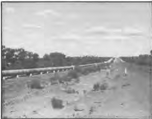
The water pipeline to Kalgoorlie.
