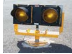
Elevated Runway Guard Light
