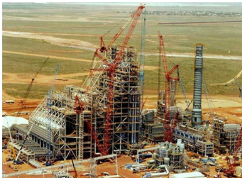
Figure 1: BHP HBI Project during construction
