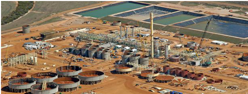
Figure 3: Ravensthorpe Nickel Concentrator during construction
