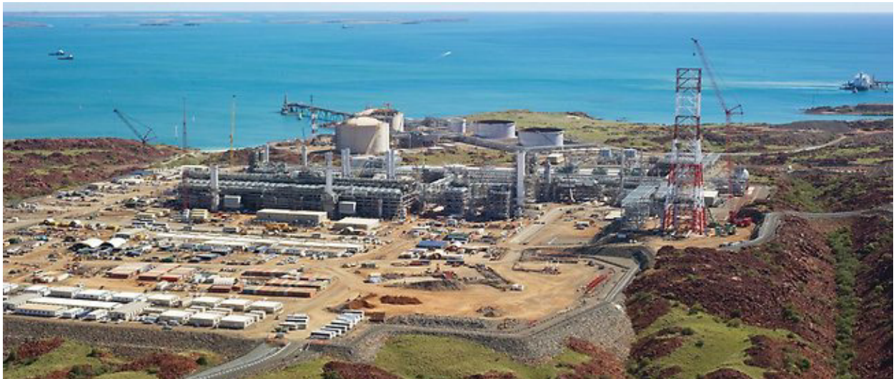
Figure 6: Pluto LNG Plant nearing completion
