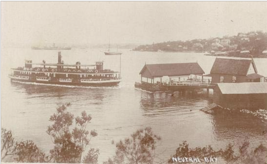
FIGURE 2 • Neutral Bay wharf; note timber pontoon and single working face of the wharf, 1927 . Source: NSC Stanton Library.
