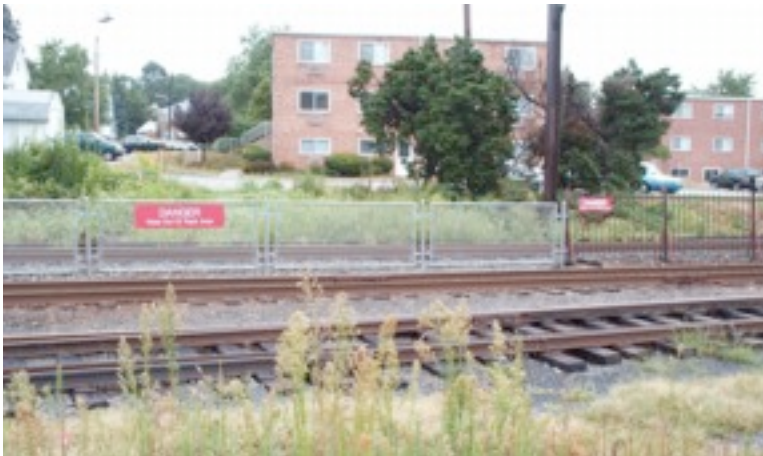
This new fence at Glenside station is keeping passengers from crossing the tracks illegally photo: Matthew Mitchell
