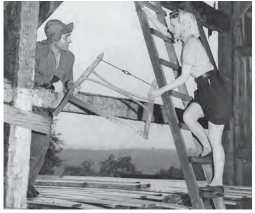
Esther Murphy and Alexander Maissel in June 1947 working on the Playhouse.
