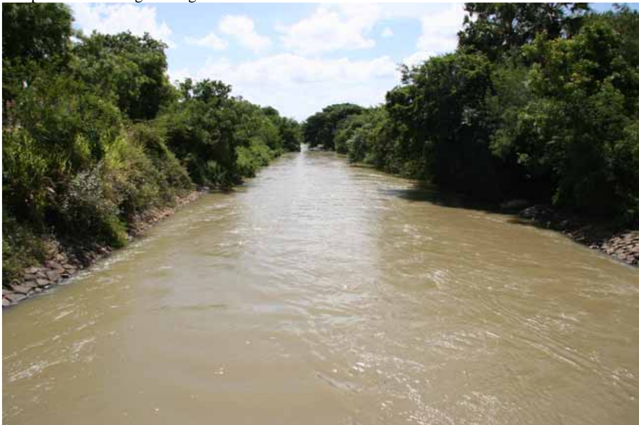
Photo 6 A recent feeder canal that runs close to the ancient feeder canal. The velocity is much higher in the recent construction compared to the ancient one. The high embankments isolate the canal from the intermediate runoff.
