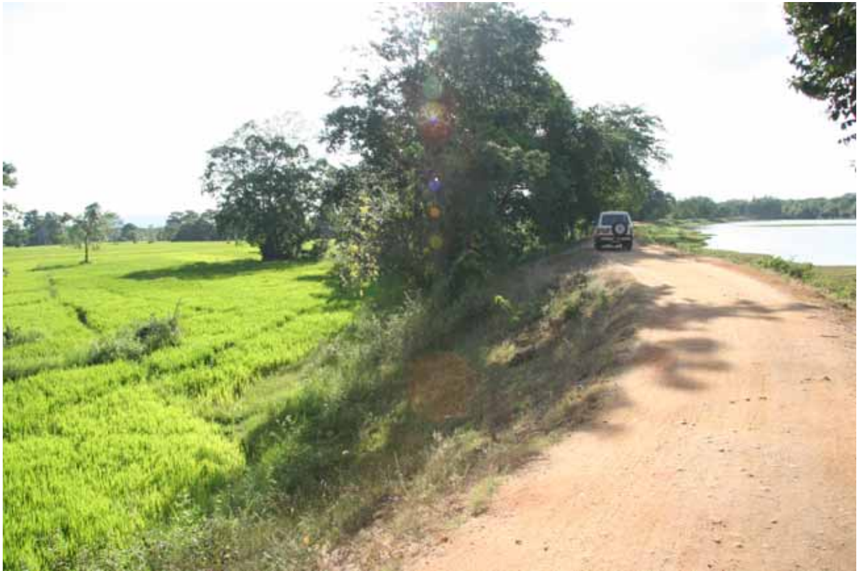
Photo 3 The length of a an embankment of a tank could vary from few 100 s of meters to 10s of kilometres .
