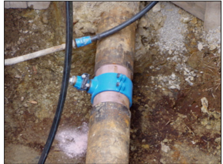
T-connection with saddle coupler
