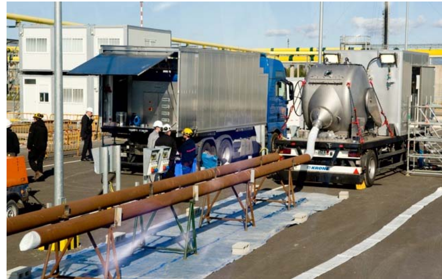
Pressure drum installation and steam equipment
