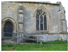
tracery typical of the Decorated period but the glass is of course much later. Also on this wall between the west end and the north transept are two further buttresses dating from the  $15^{\text{th}}$  century. We believe that this indicates that the clerestory was added in the  $15^{\text{th}}$  century when these buttresses were built. The west end already had adequate buttressing.
