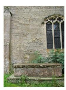
The chancel north wall is one of the most interesting puzzles in the church and it is evident that it also has been increased in height at some stage - the buttresses would suggest sometime in the 14<sup>th</sup> century. The buttresses would have been necessary as the wall was pierced to accommodate larger windows.
