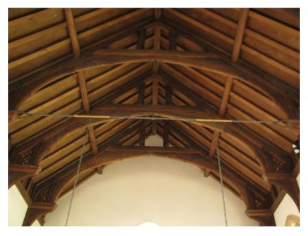
Looking upwards we see a Victorian roof that is of hammer beam construction with a deal of additional decorative work.
