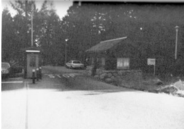
Illustration 207. South Entrance kiosk and office. Photo by Gary Higgins, 1984.
