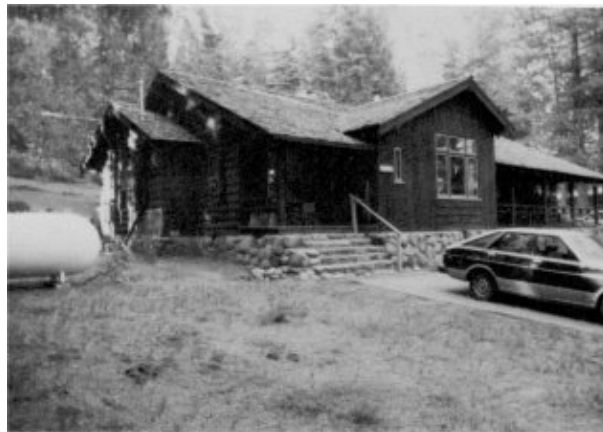
Illustrations 212-14. Utility building, Yosemite Valley maintenance yard. Notice similarities in style between this building and the valley power plant. Photos by Gary Higgins and Robert C. Pavlik, 1984.
