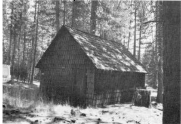
Illustration 195. Wawona barn, utility area.
