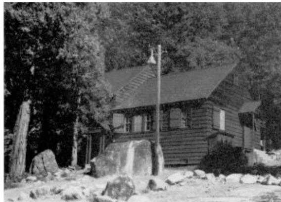
Illustration 250. Lake Eleanor dormitory built by City of San Francisco. Photos by Robert C. Pavlik, 1984.
