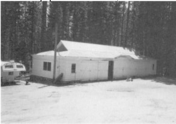
Illustration 194. Wawona equipment shed #4052, to southwest.
