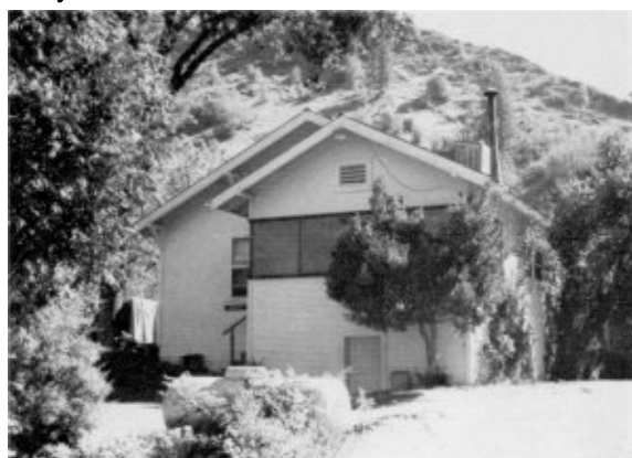
Illustrations 127-28. Rancheria Flat houses built by National Lead Company. Photos by Robert C. Pavlik, 1985.
