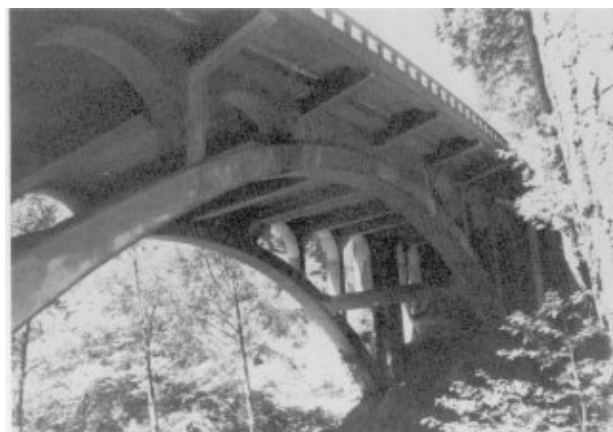
Illustration 158. Road bridge over Tuolumne River.
