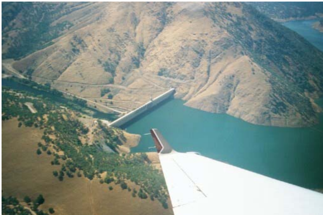
Pine Flat Dam, view N, 5/29/02
