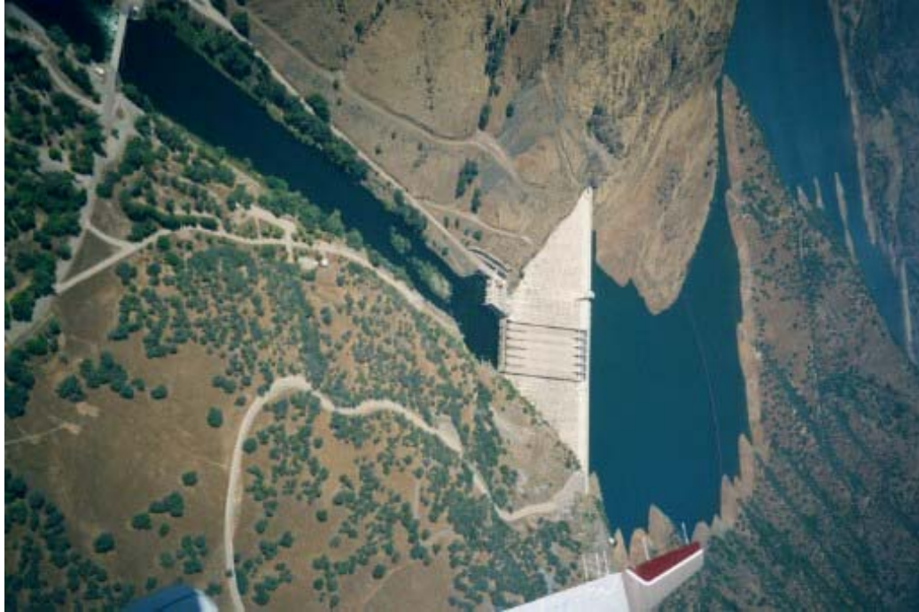
Pine Flat Dam, view NE, 5/29/02
