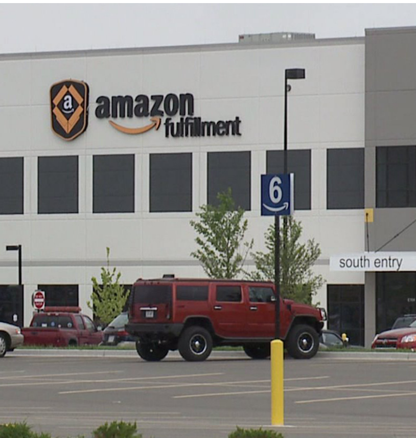
Amazon secured $27.3 million in public subsidies from state and local officials to build this fulfillment center in Kenosha, Wisconsin.
