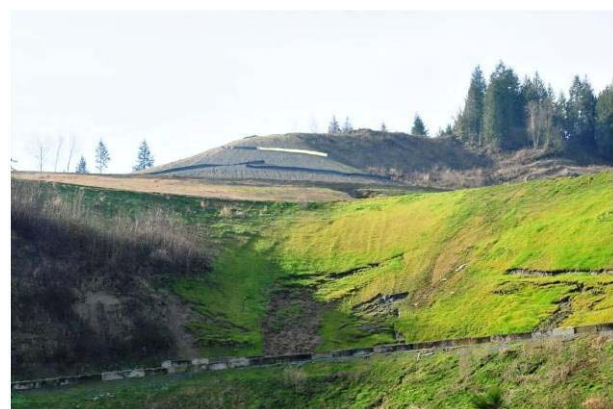
Hillside development with signs of unchecked erosion.
