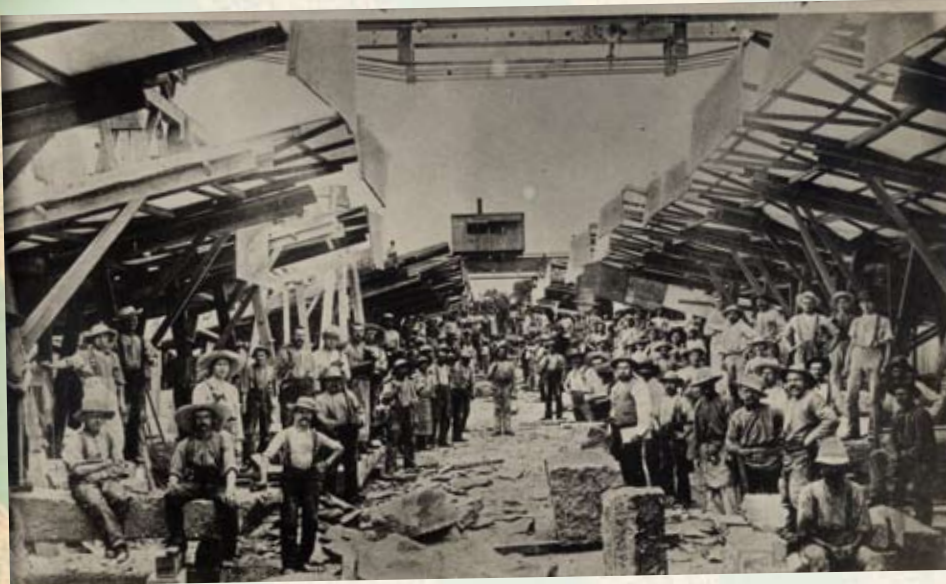
Work for construction of new Capitol, Scottish stonecutters in granite yard, Burnet, Texas, 1884. Photographer: N.M. Wilcox. (Prints and Photographs Collections, Texas State Library and Archives Commission)
