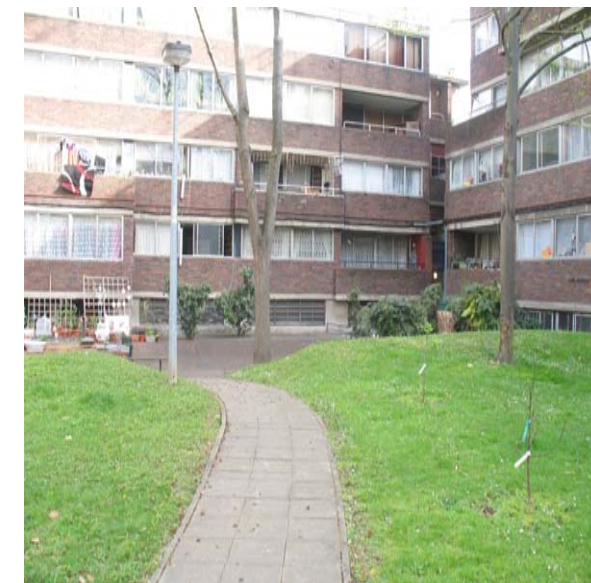
41 Louvred vents to existing garages. Baseline windows can be seen to the right.
