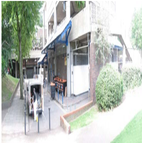
5 Service Access to east side of tower
