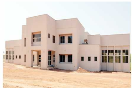
Completed building at Bayero University, Kano
