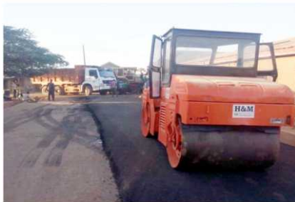
Construction of Roads, at Bayero University, Kano
