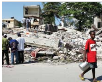
People sift through the rubble in downtown Port-au-Prince, seeking to salvage usable building materials and personal objects.
