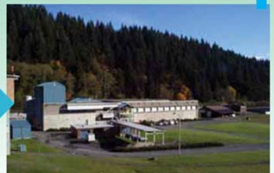
Drinking water treatment facility
