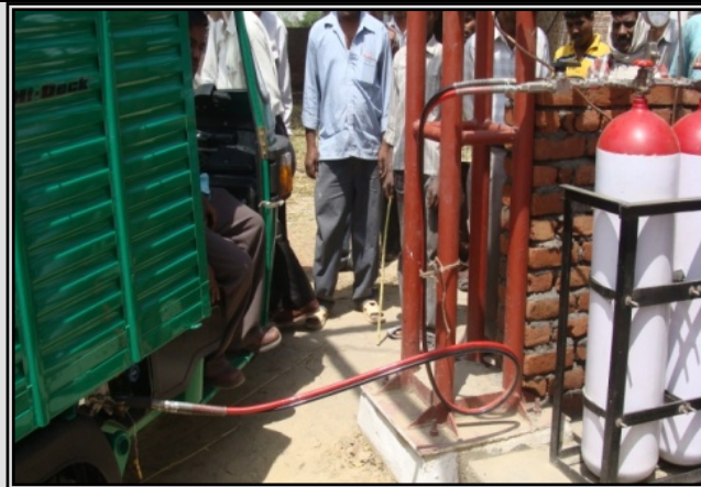
Biogas High Pressure Cylinder and Compressor
