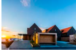
Residential construction - Stavanger/Myklebust, Norway
