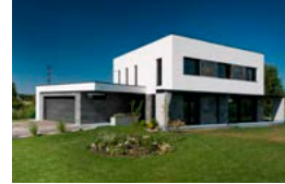
Private residential construction - Warsaw/Zielonki, Poland
