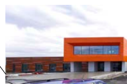
Commercial construction (offices) - Reci, Romania]
