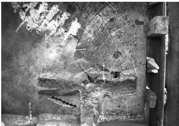
Figure 5. Metal stitching castings
