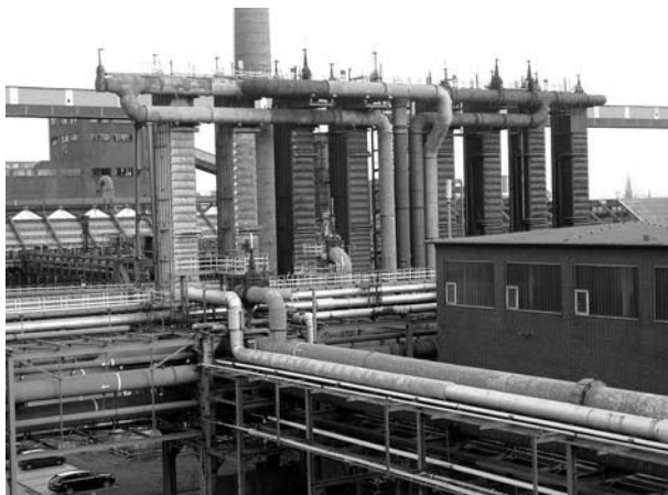
Figure 4. Details from Kokerei Zollverein (white side) showing pipeline bridges, buildings and tube cooler units in the background.
