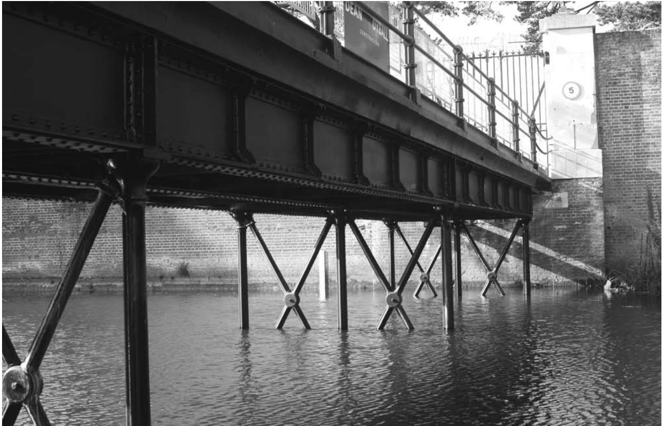
Figure 9. Fort Brockhurst Bridge – fully conserved and rebuilt
