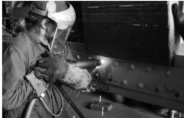
Figure 7. Re-riveting an I-beam
