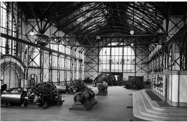
Fig 6: Interior space of the engine house with air compressors and winding machines, early 20th century (Siemens Archives, Munic)
