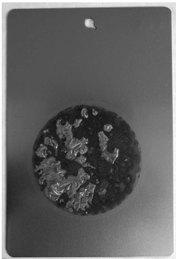
Figure 6: Panel coated with Poligen ES91009 after 24 hours in contact with 0.5M sodium chloride solution. The circle shows the area exposed to solution while in the electrochemical cell. Bare metal is visible where the panel has lifted
