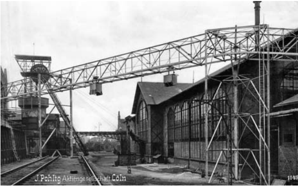
Fig 5: South façade of the engine house. An elevated monorail connects the coal washery and the boiler house, early 20th century (Bergbau-Archiv, Bochum)
