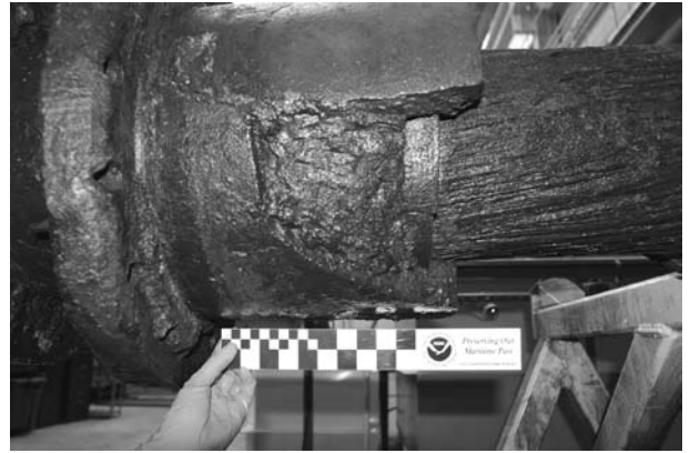
Figure 9: Packing material and aft packing ring revealed by crack in cast iron.
