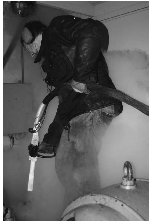
Figure 3. Abrasive blasting with dry ice pellets (09.08 Beck)
