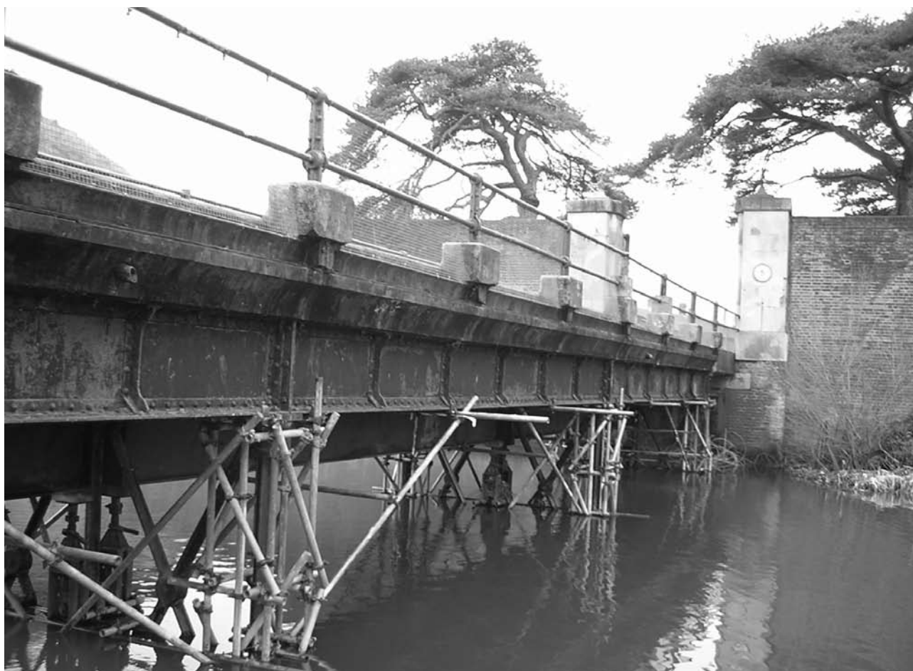
Figure 2. Fort Brockhurst Bridge before conservation
