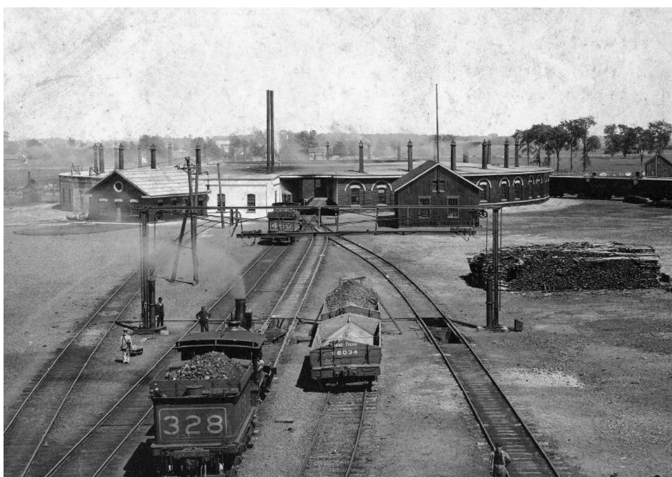
ABOVE: ROUNDHOUSE IN YARD 2, CIRCA 1900. TOP: ENGINE ON TURNTABLE IN ROUNDHOUSE, CIRCA 1900.
