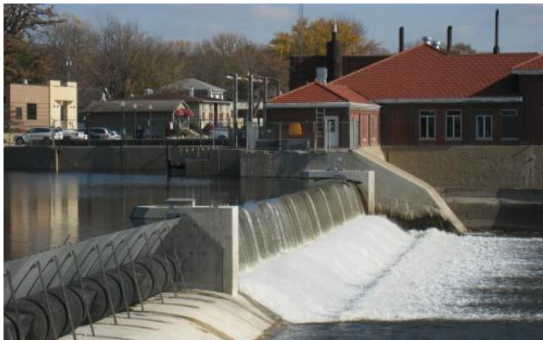
Figure 2.11 Inflatable Crest Gates (Representative Diagrams, For Illustration)
