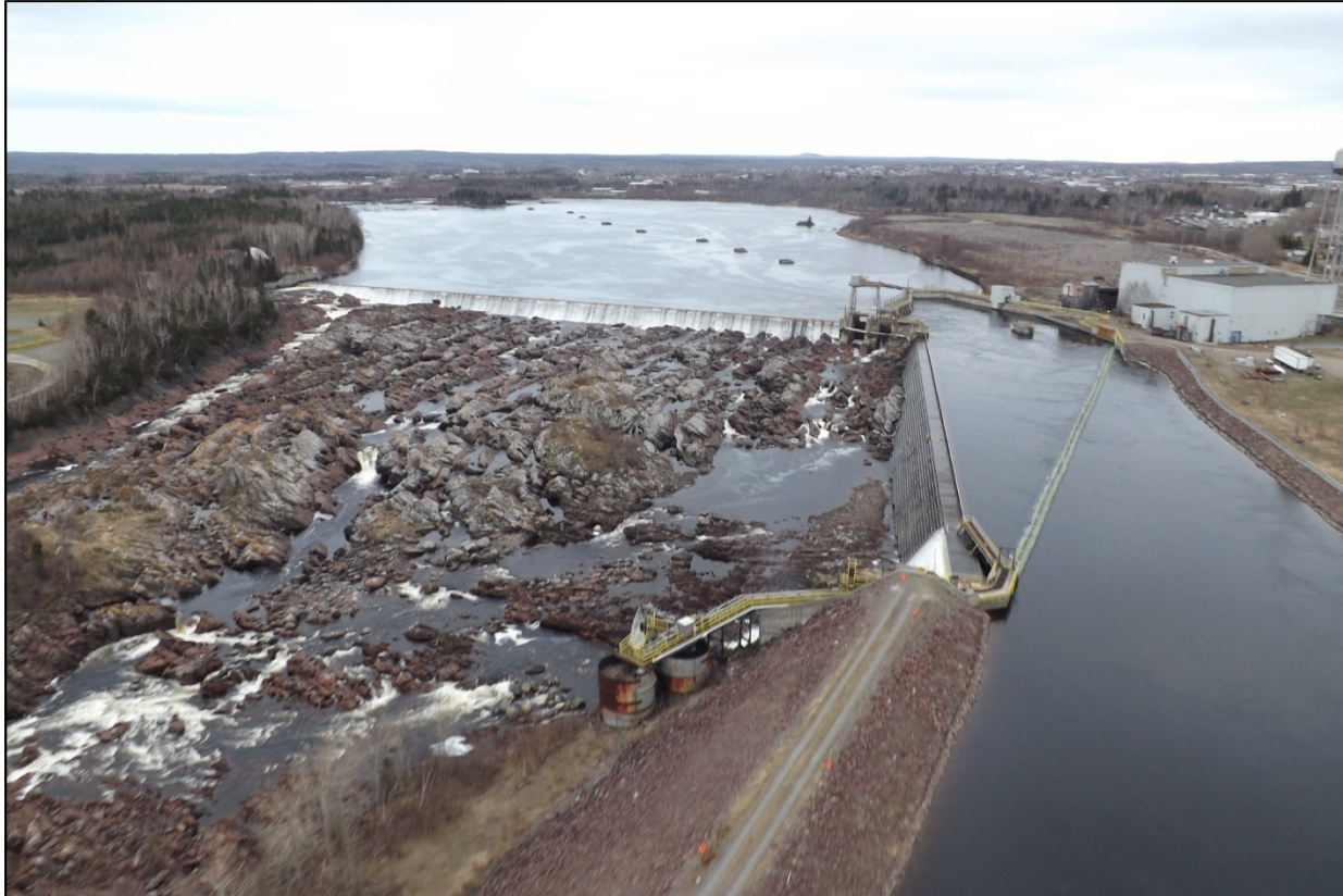
Figure 2.4 Grand Falls Generating Facility (Photographs)
