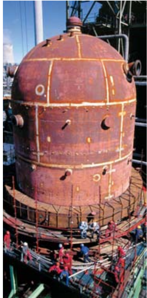
Assembling a SAS reactor – there was little room to move
