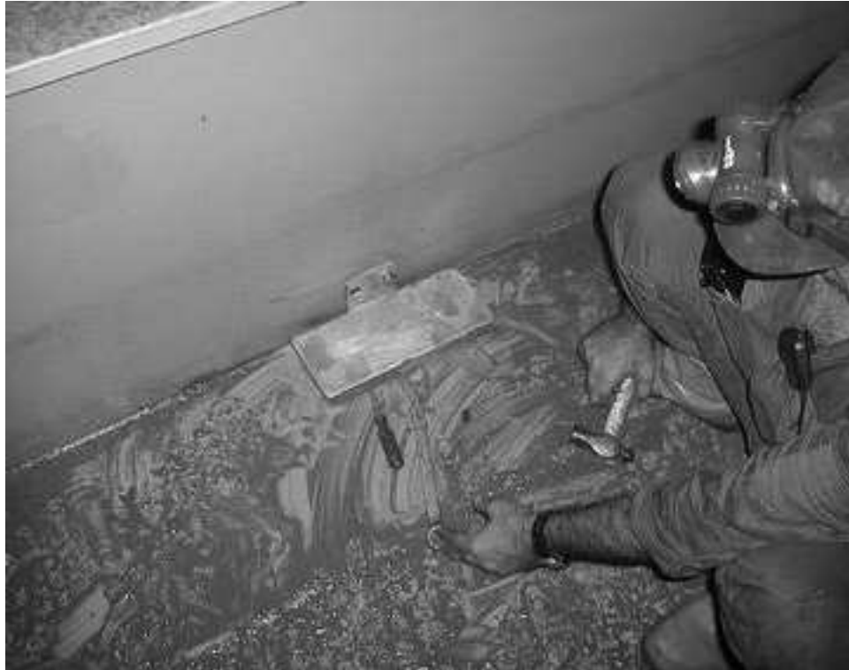
Figure A.1: Installation of Tsevas Pitguard
