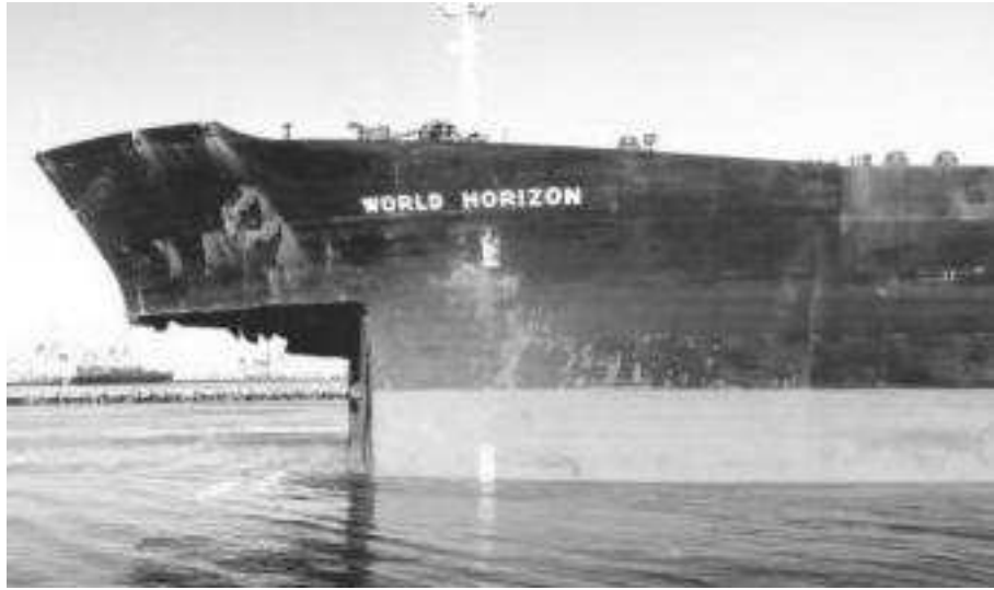
Figure 2.8: World Horizon after “freak wave” removed forepeak tank. This wave was able to excise only the forepeak tank with almost surgical precision. The true cause was that this segregated ballast tank was very badly corroded. The surrounding spaces were not. Spill was about 850 kiloliters. Source: University of Capetown.
