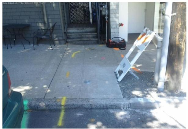
Figure 2 – Locating Inc. documented completed locates on July 14, 2016 at 2:32 p.m. Above is the sidewalk taken facing north from NW Glisan prior to PGE and Loy Clark Pipeline opening an excavation in conjunction with city permit #65193. The natural gas service line is clearly visible showing a complete field location of the service line between 500 NW 23<sup>rd</sup> Avenue (building on the left) and 2281 NW Glisan Street (building on the right).
