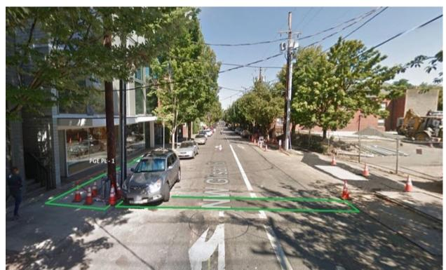
Figure 3 – Google Street view facing East on NW Glisan – Shows PGE PL-1, risers installed by Loy Clark on the *North* side of Glisan, Restored street and sidewalk surfaces (highlighted in green) across NW Glisan Street and from PL-1 to PGE Vault – 95 in front of 2281 NW Glisan Street.
