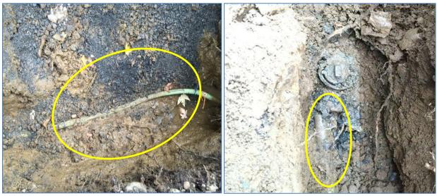
Figure 6 - Damaged service line
