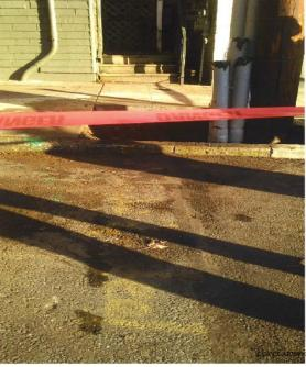
Figures 4 and 5 – Photographs obtained from Oregon OSHA, taken by Loy Clark Pipeline after striking the Natural Gas Service line. The valve lid (also in Figure 2) is between two faded markings. Loy Clark Pipeline did not have clear visible field locations in order to identify the presence and direction of the natural gas service line beneath restored section of sidewalk.
