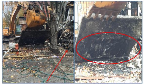
Figure 8 – Sidewalk removal revealed vault in the right-of-way Figure 9 – Bottom of sidewalk was a ceiling surface of vault
