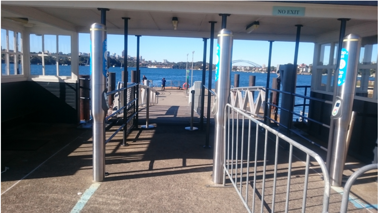
Plate 11 Former security box, known as the Bundy Office, looking east down the gangway to the pontoon (RPS, 2015).
