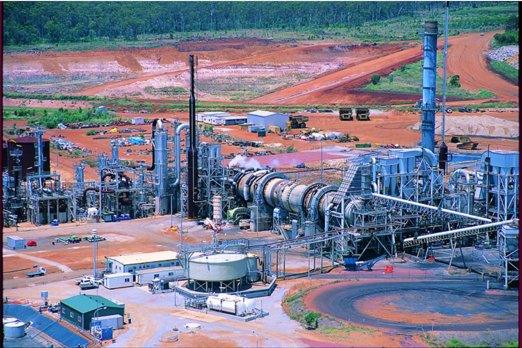
ATP Processor Retort Technology at Stuart Oil Shale Facility, Queensland, Australia (This is a demonstration-scale [4,800-bbl/day] oil shale facility. A portion of the oil shale mining area is visible in background. Photo courtesy of Queensland Energy Resources Limited, Queensland, Australia, and UMATAC Industrial Processes, Calgary, Alberta, Canada. Reprinted with permission.)
