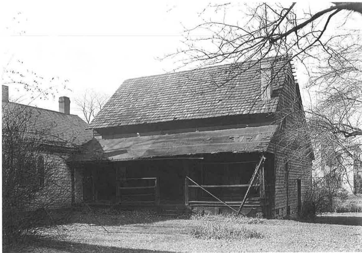
Image 6. View of the Magazine, looking southwest, 1936.
