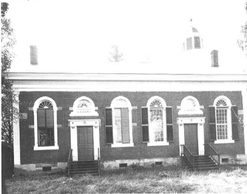
Image 11. View of Meeting House, looking south, 1890s.
