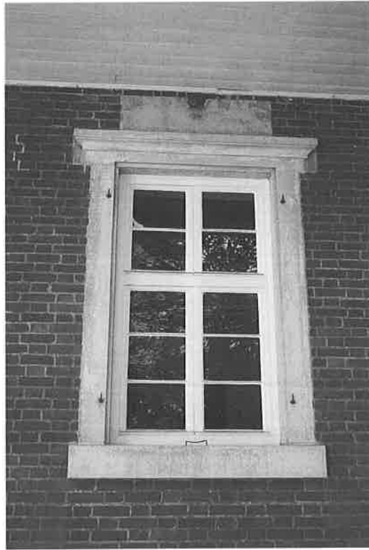
Image 11. Detail of stone window surround at the Number One House.
