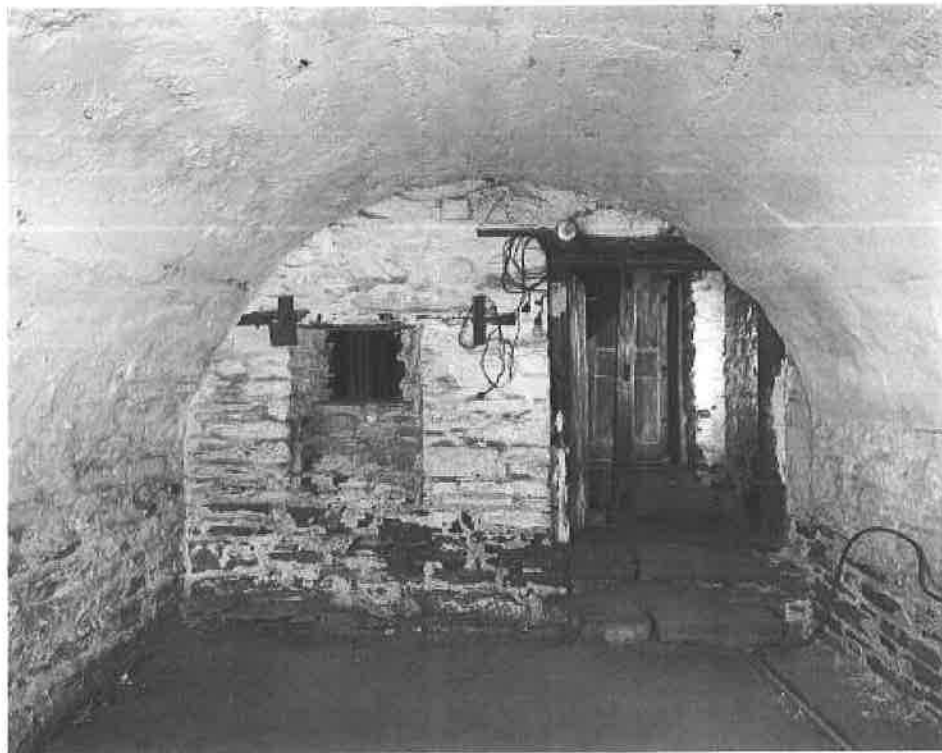
Image 2. View of the vaulted cellar of the Schaeffer House (1736), Schaefferstown, Pennsylvania, 1997.
