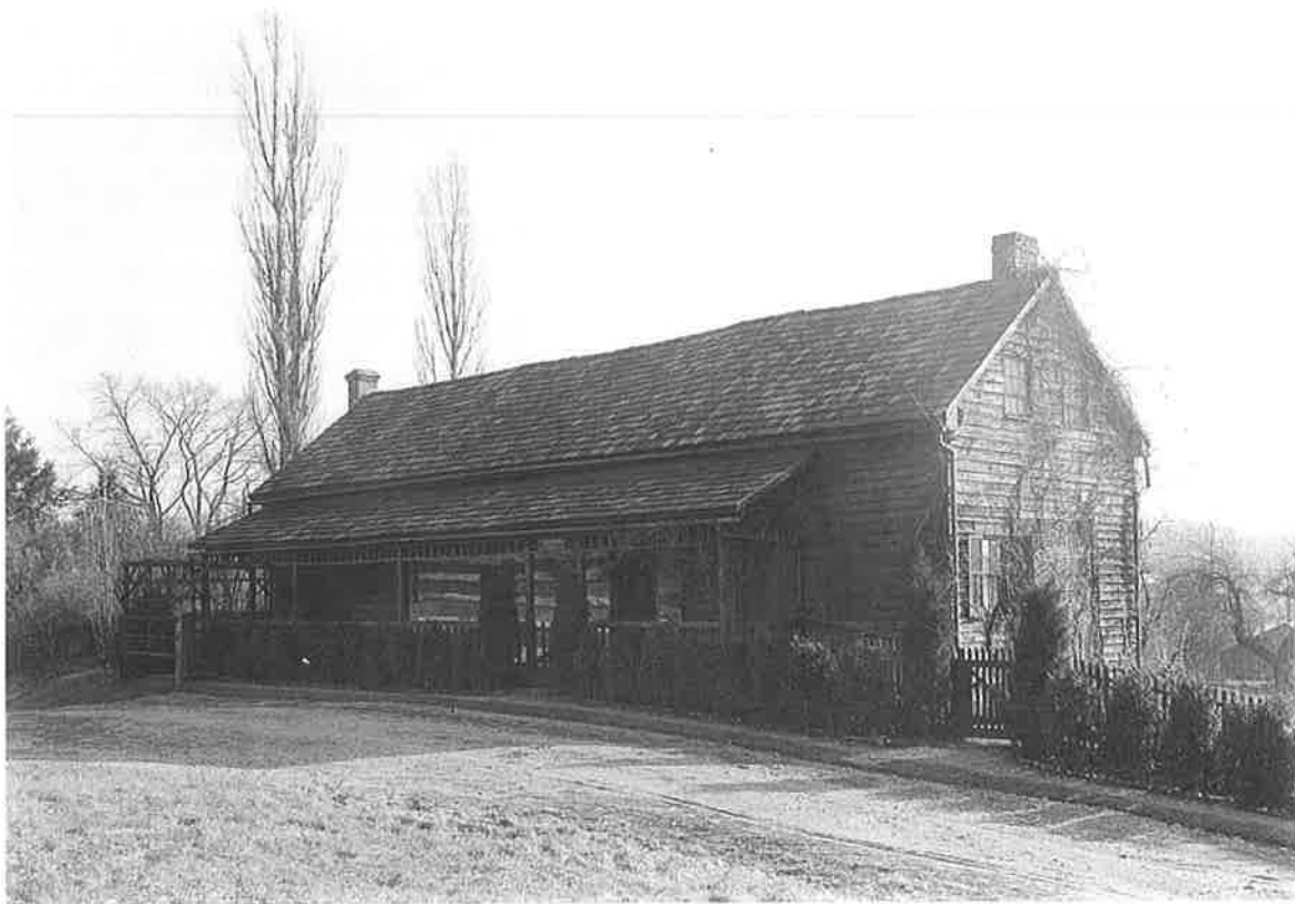
Image 14. View of Print Shop (#16), looking southeast, 1936.
