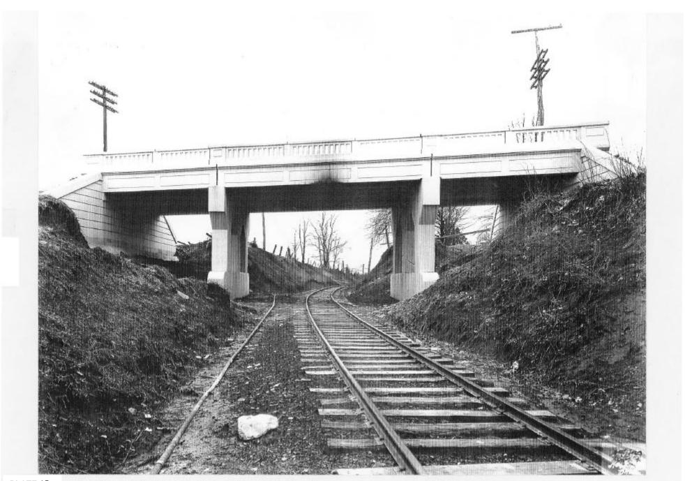
PLATE 15: Typical Concrete Multiple-Span Beam Bridge: Bridge Crossing Railroad Tracks at Fallston
