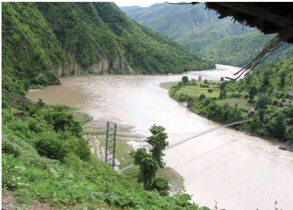
The Bridge over the Arun River at Anterighat
