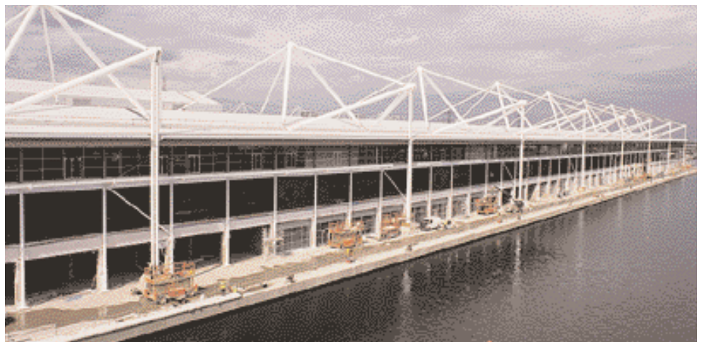
The specified live load for the exhibition floor is very high, 20 kN/m 2 on average, thus facilitating heavy equipment exhibitions.
