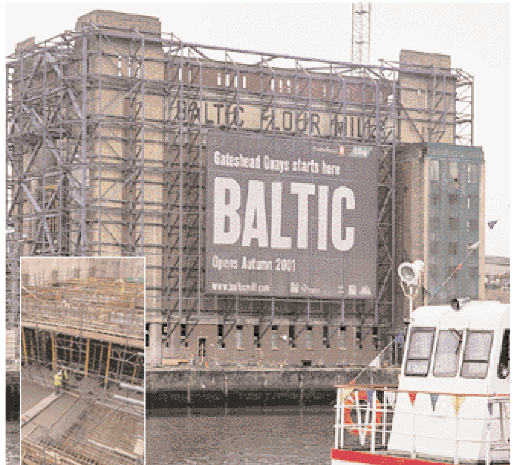
To accommodate the art centre, the Baltic flour mill structure is transformed to receive three RC floors and three RC mezzanines.
