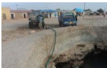
The main water well for drinking
