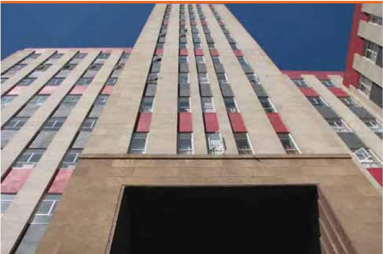
International Housing Solutions building upgrade in Johannesburg
