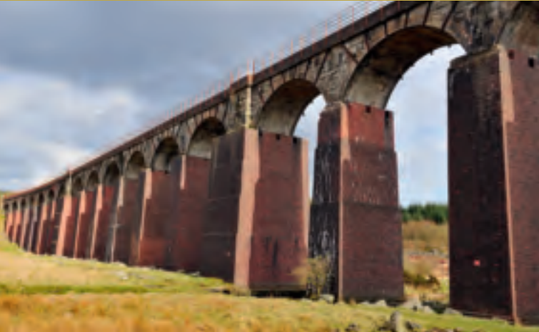
The old railway viaduct at Gatehouse of Fleet
