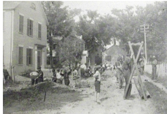
Figure 17 Construction on Church St in Mattapoissett [7]
