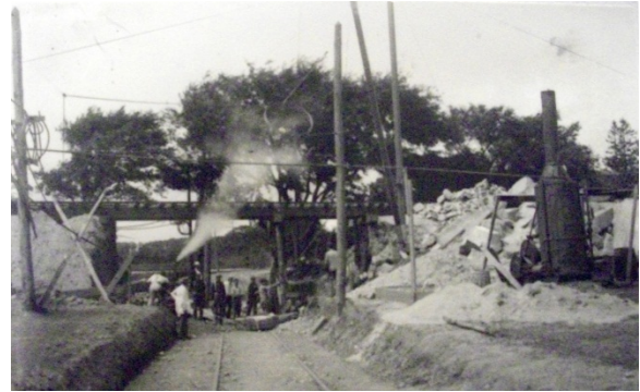
Figure 16 RR Underpass at Mattapoissett [7]
