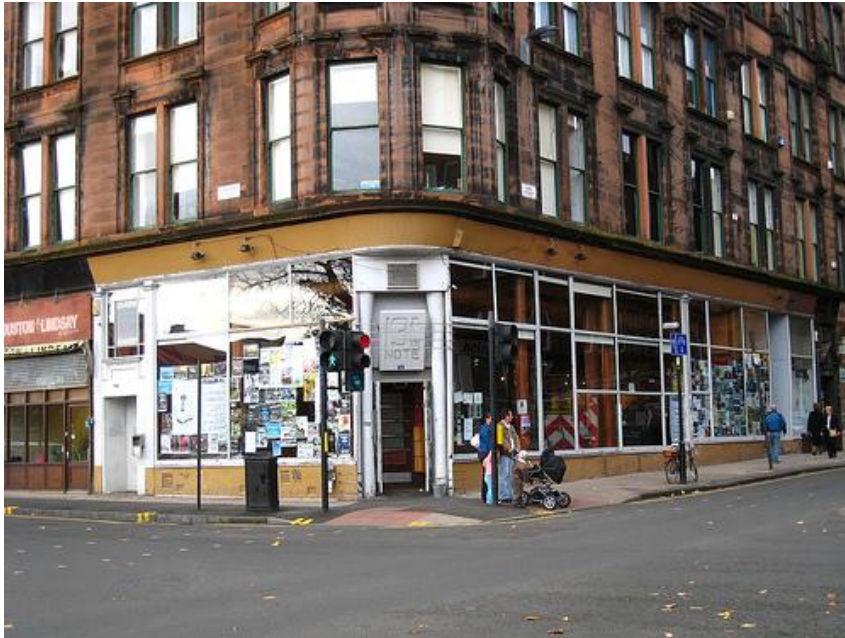
Fig 12 The exterior of The 13 th Note in Glasgow.
