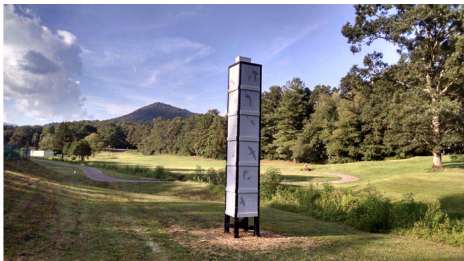
One of two newly constructed chimney swift towers; Chris Kelly.
