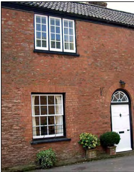
Fig.20 Sash, casement windows and fanlight at Redstone Cottage (Zone 1).
