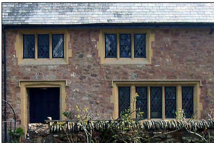
Fig. 18 Ham stone dressings and exposed rubble sandstone at Cridlands (Zone 1).
