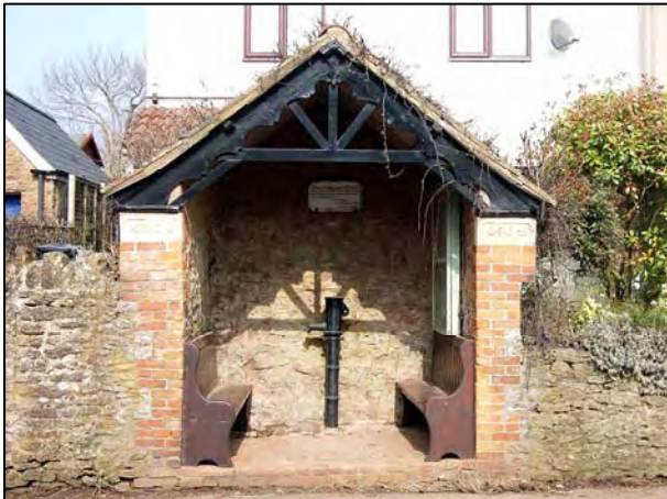
Fig.26 Pump house on the main street (Zone 1).
