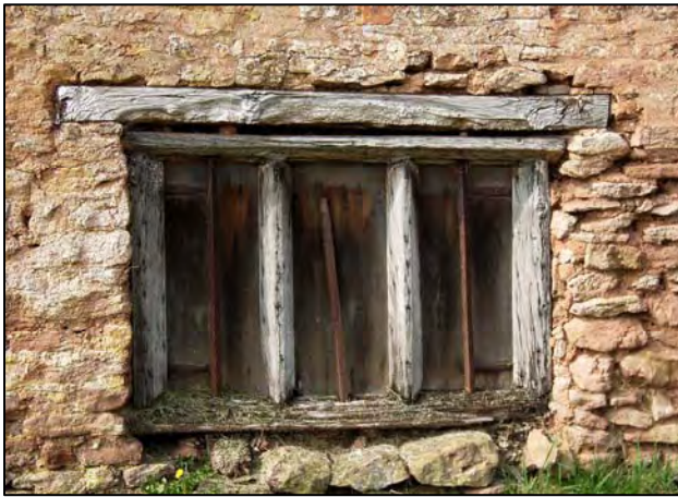
Fig.21 The 17 th -century timber mullioned window at Hill's Farm (Zone 1).
