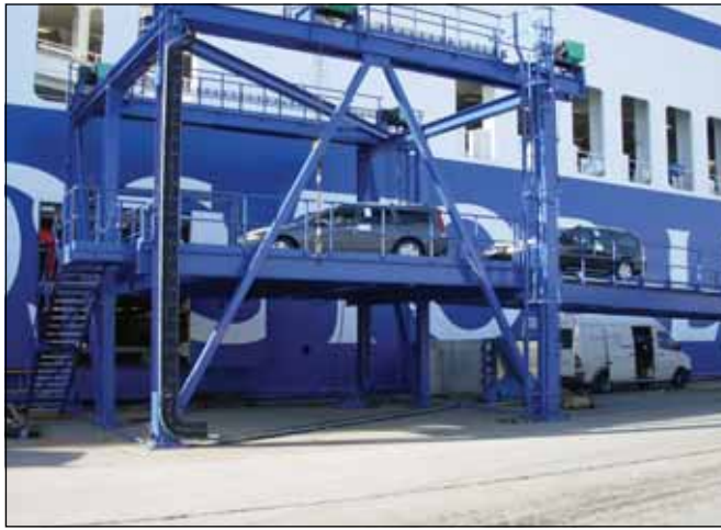
The new ramp at the Mercatordok multimodal facility was designed by Antwerp-based Catracom
