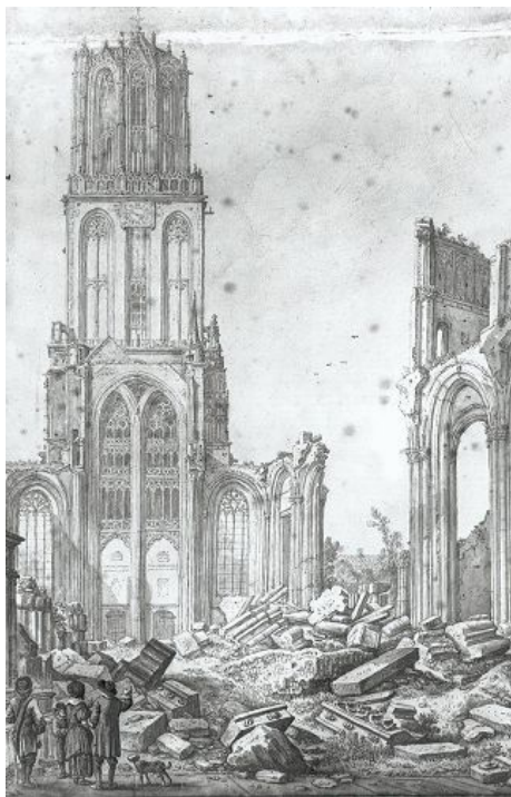
Figure 1: A tornado caused the collapse of the nave of the dom church of Utrecht in 1674. The nave was never rebuild and only the tower remains to this day. Source: Het Utrechts Archief: Drawings by Herman Saftleven.
