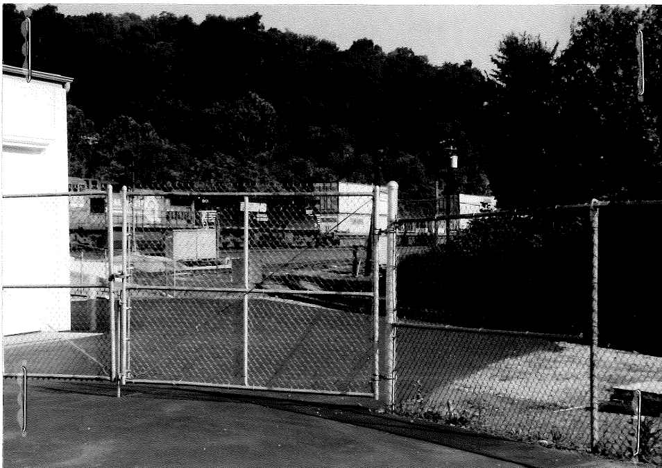
Photograph 3: Looking northwest at junction of Norfolk Southern Railroad and Turtle Creek Industrial Railroad.
