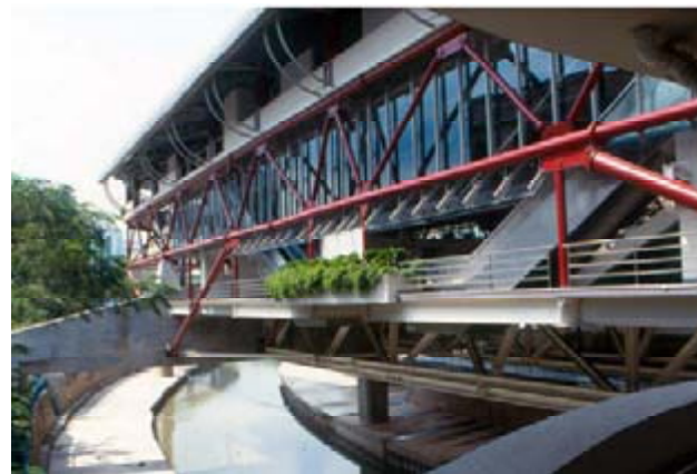
PWTC Station- View towards Gombak River
