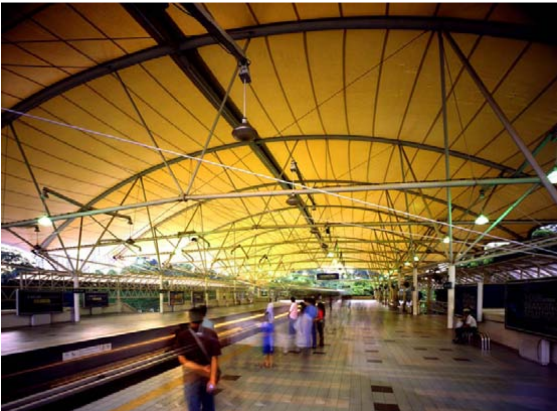
Bukit Jalil station, platforms and canopy roof.
