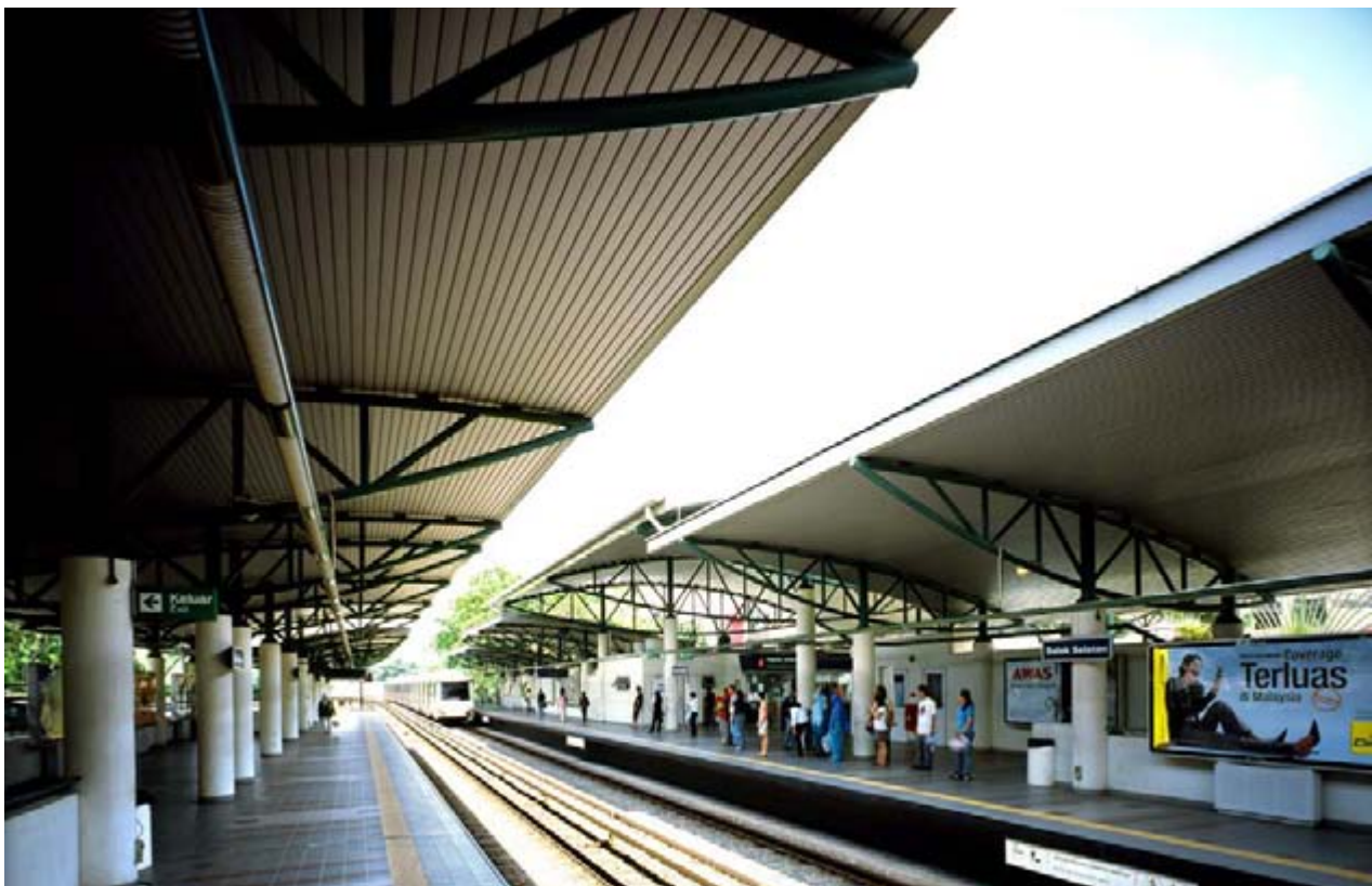
Salak Selatan station platforms.
