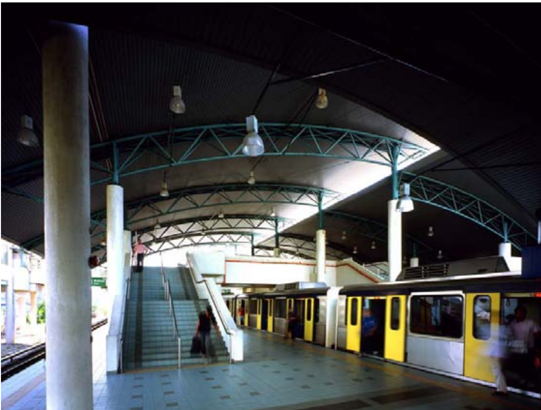
Tasik Selatan station platforms.
