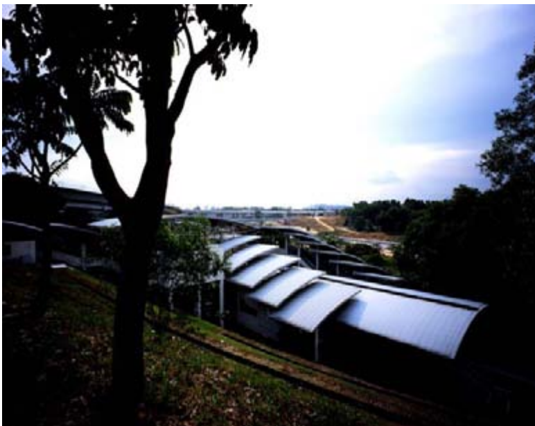
Sri Petaling station, exterior view.
