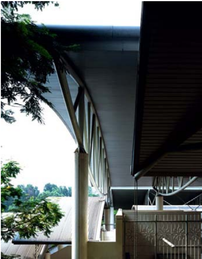
Sri Petaling station, curved roof supported by steel “finger” trusses.
