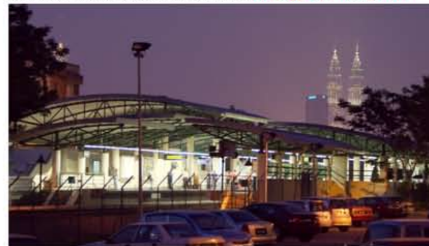
Salak Selatan Station
