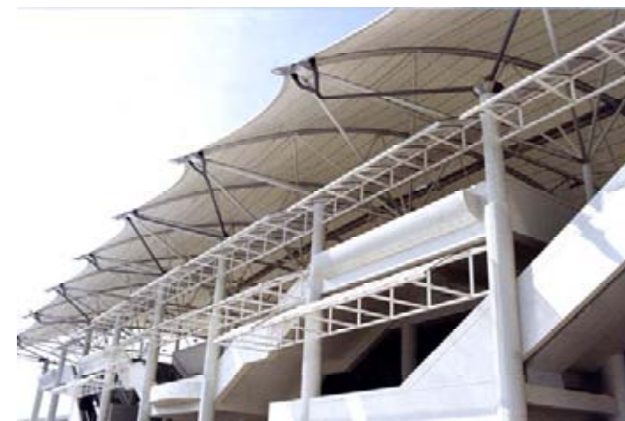
Bukit Jalil- View from approach road
