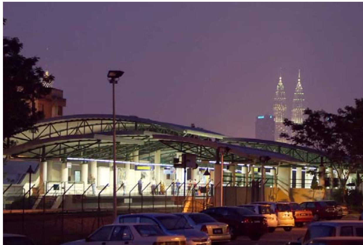
Salak Selatan Station- Night scene
