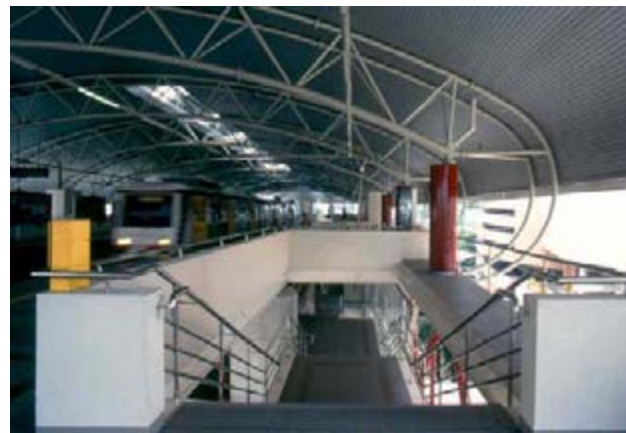
PWTC Station- Interior view
