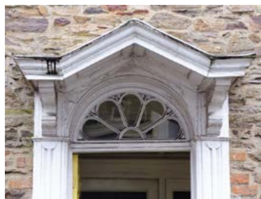
Fig. 77 Fanlight at Billbower House
