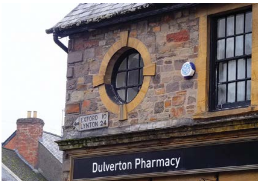
Fig. 33 First floor roundel window to Dulverton Pharmacy.
