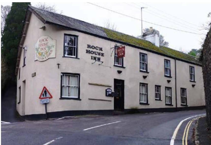
Fig. 60 Rock House Inn, top of Vicarage Hill
