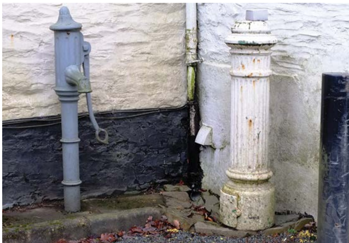
Fig. 81 Bollard and hand pump at Northmoor Road
