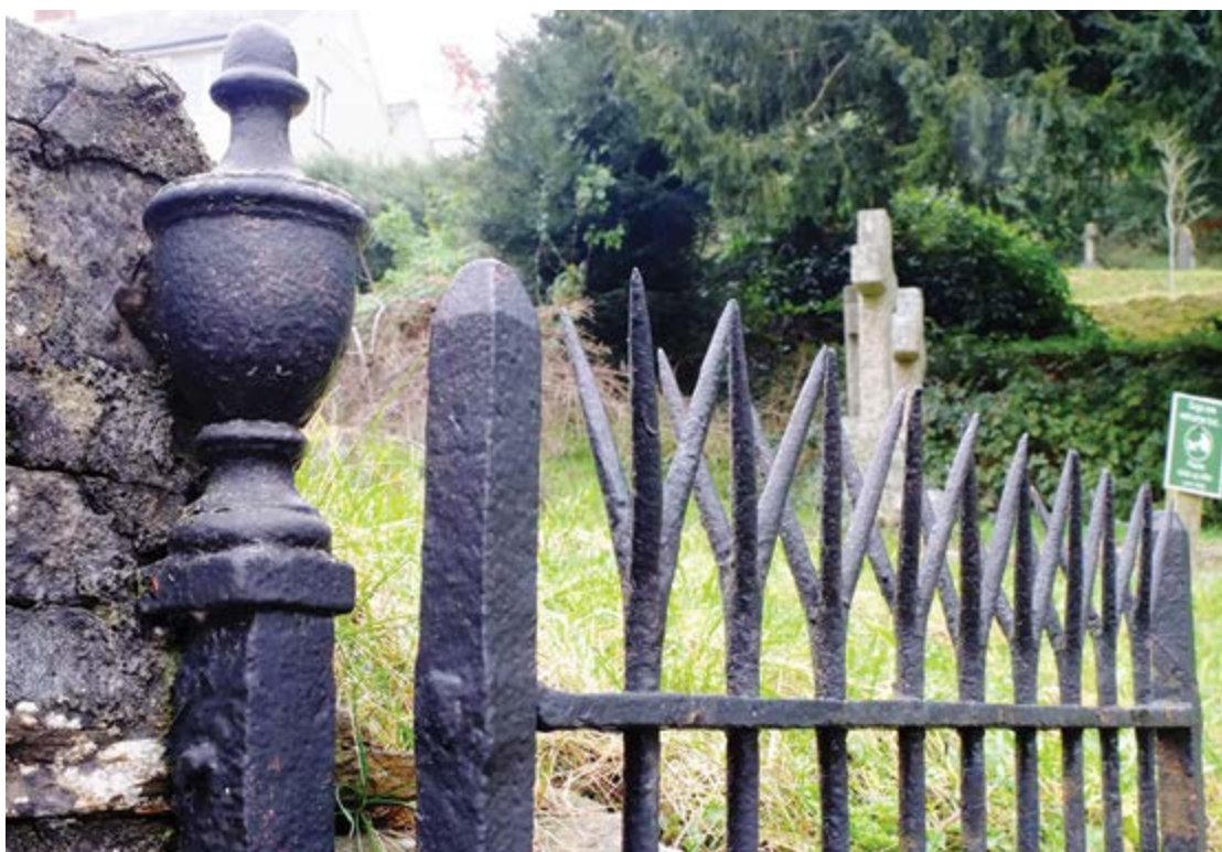
Fig. 79 Part of the ironwork surrounding the church.
