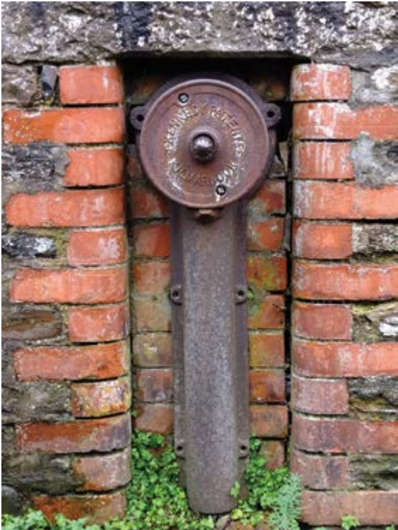
Fig. 82 Water hydrant, Church Lane
