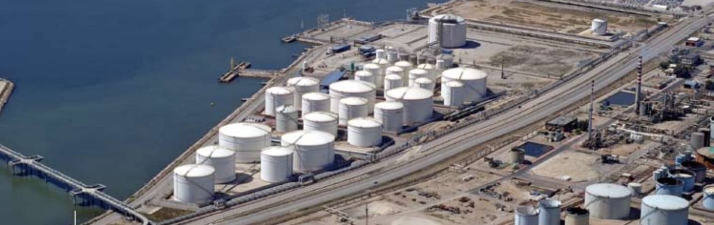
TAPP AIE - oil products terminal, Port of Tarragona, BASF and Dow
