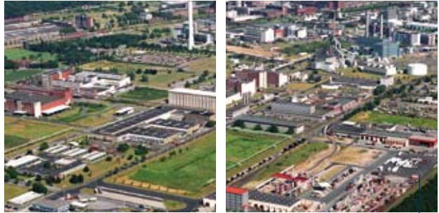
Chemical plant, Dormagen, Bayer
