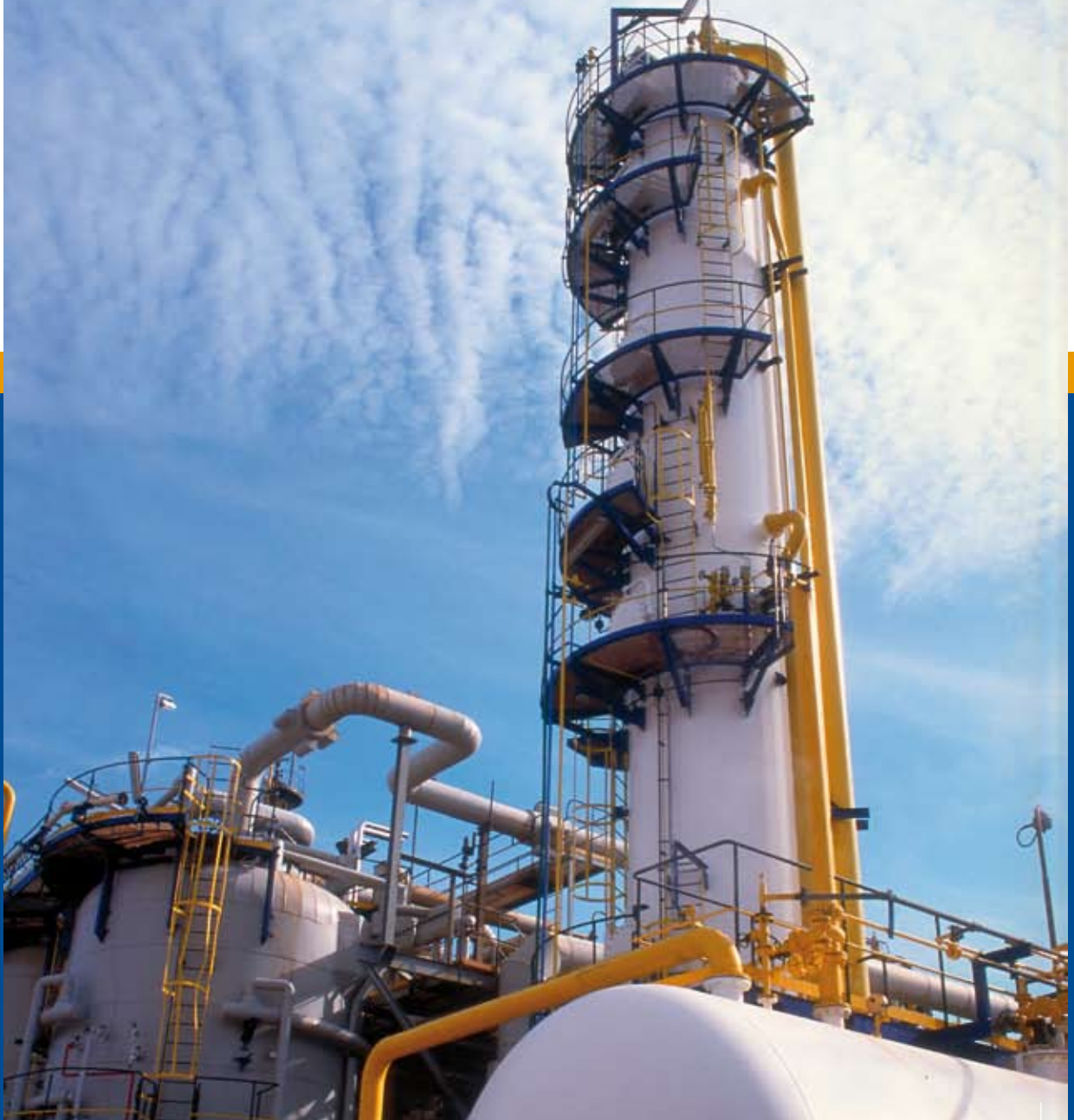
Towers of distillation for the production of VCM at plant, Vila-Seca - Tarragona, Ercros
