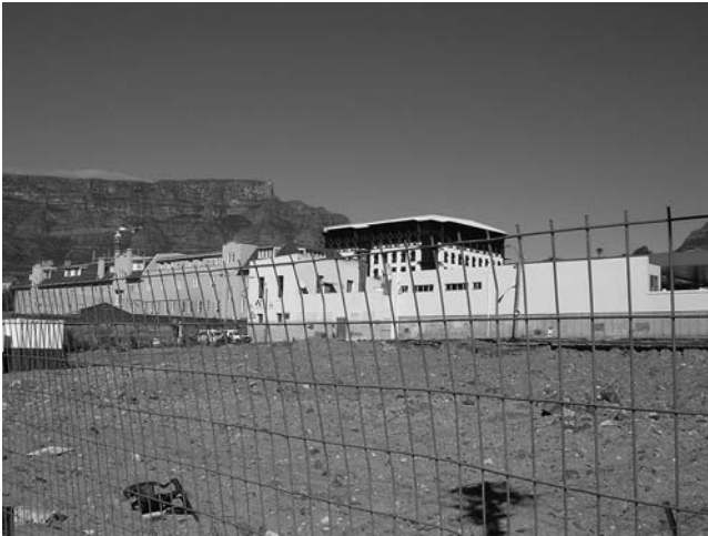
Figure 5.2 Prestwich Place as construction site in the new Cape Town. Photograph by J. Jonker, 2006.
