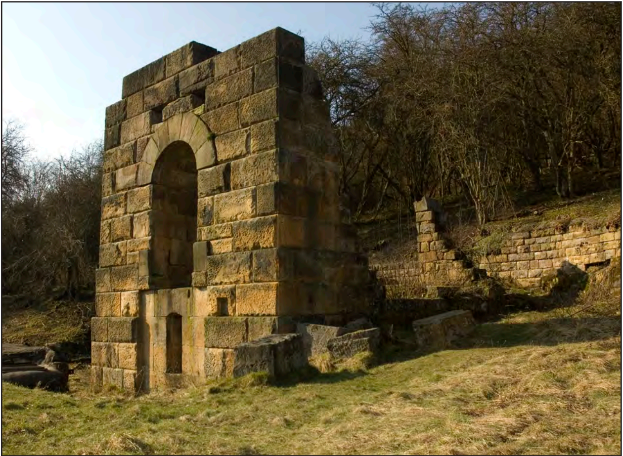
Plate 1: The ruined pumping engine house at Watt's Engine (Site 199) is one of the little visited gems that remain from the Peak District's historic lead mining industry.
