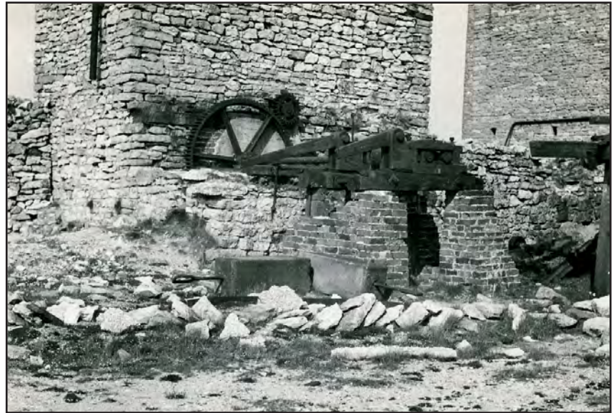
Plate 37: Site 129: The rolls crushers and weights at Magpie Mine in the earlier-20th century, with their small engine house behind in better condition than today. No examples of rolls crushers survive today at Peak District mines.
