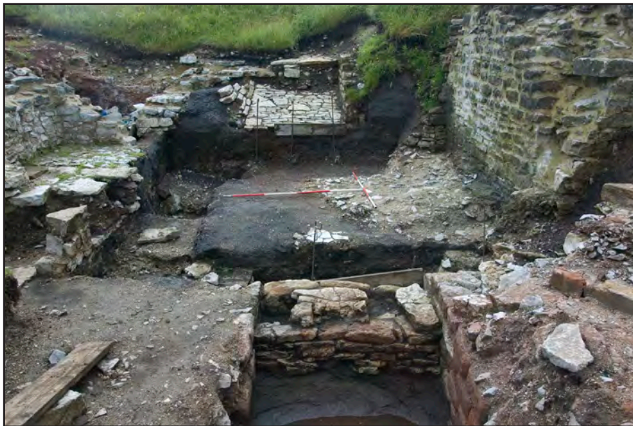
Plate 35: Site 59: The largely-removed 1794 Newcomen pumping engine house at Watergrove Mine under excavation in 2012, with coal storage hopper behind, original boiler ash pit in foreground, coe to left and later ash pit behind this. Of the features exposed, only the bob wall to right was visible before excavations started.
