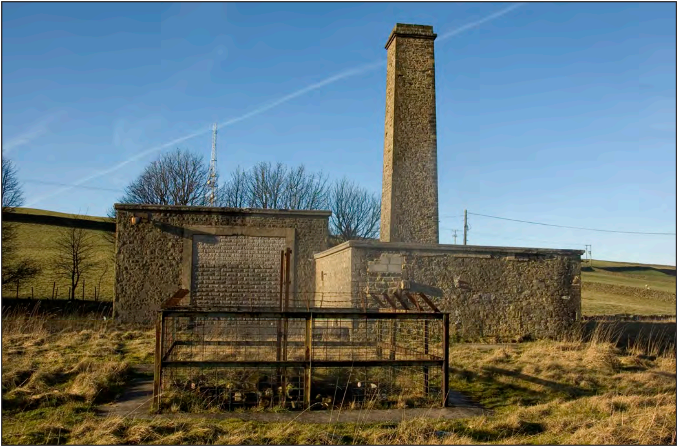
Plate 5: All that stands today on the large hillock of the once important Ladywash Mine (Site 47) is the chimney of a 19th century lead mining engine house, with more modern buildings used when the shaft was used to bring fluorspar to surface in the 20th century. The fenced shaft top is in the foreground. Archaeological remains at disused gangue mines are rare and while more modern are just as important.
